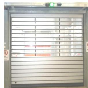
Figure 6: High-speed spiral door
