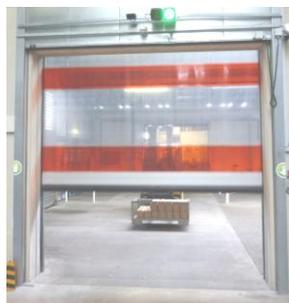
Figure 4: Flexible high-speed door
